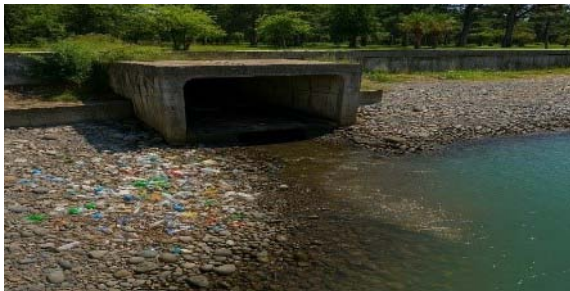
Figure 6. Stormwater Drainage Outlets near Batumi
